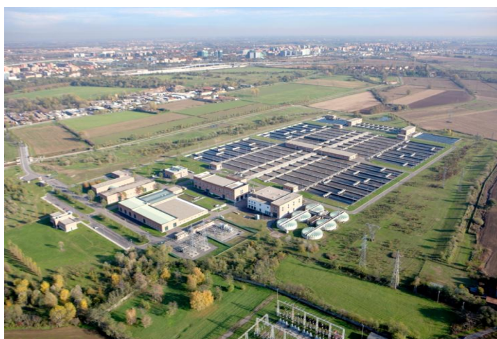
Figure 1. Aerial view of Milan Nosedo WWTP
